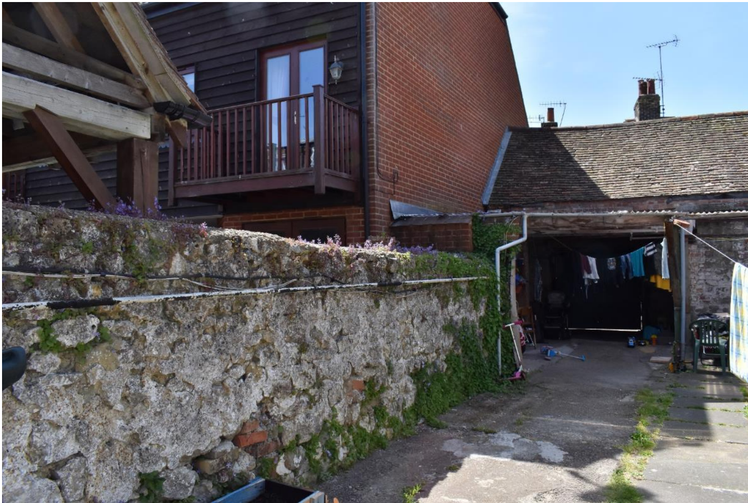
Plate 13: View of the eastern boundary (facing S)
