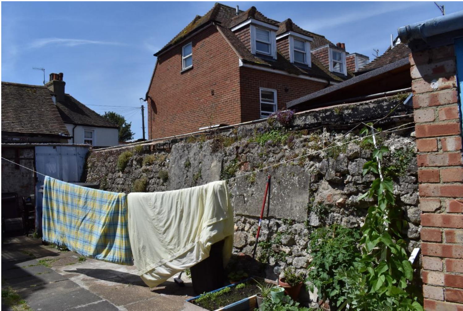
Plate 12: View of the western boundary (facing SW)
