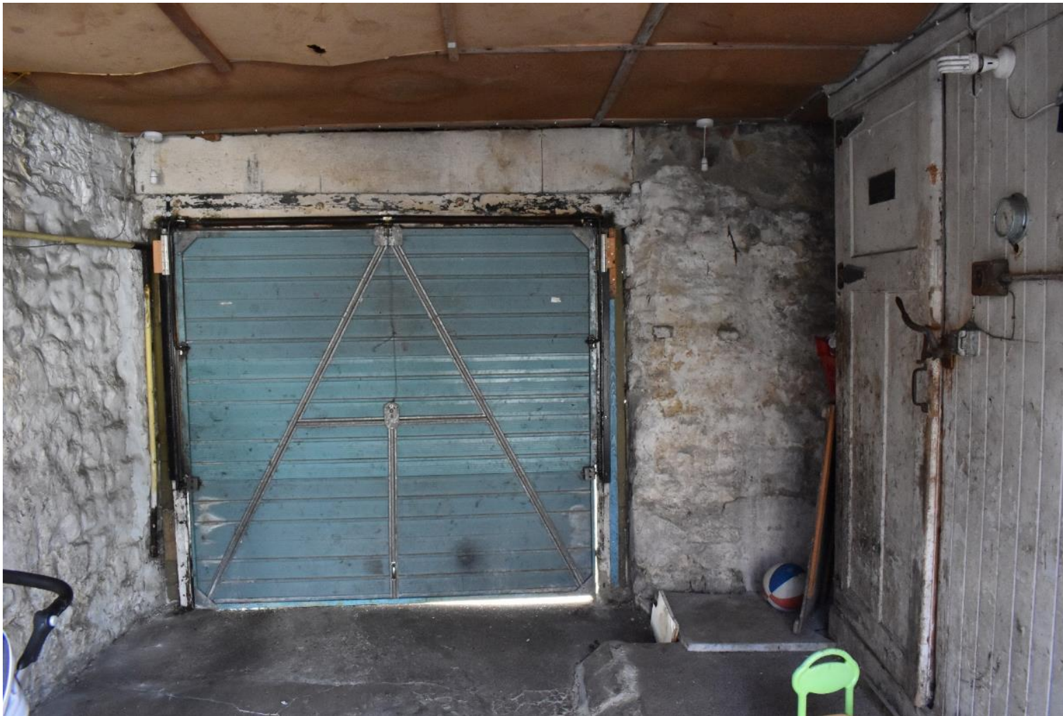
Plate 17: View of rear entrance from PDA (facing SSW)
