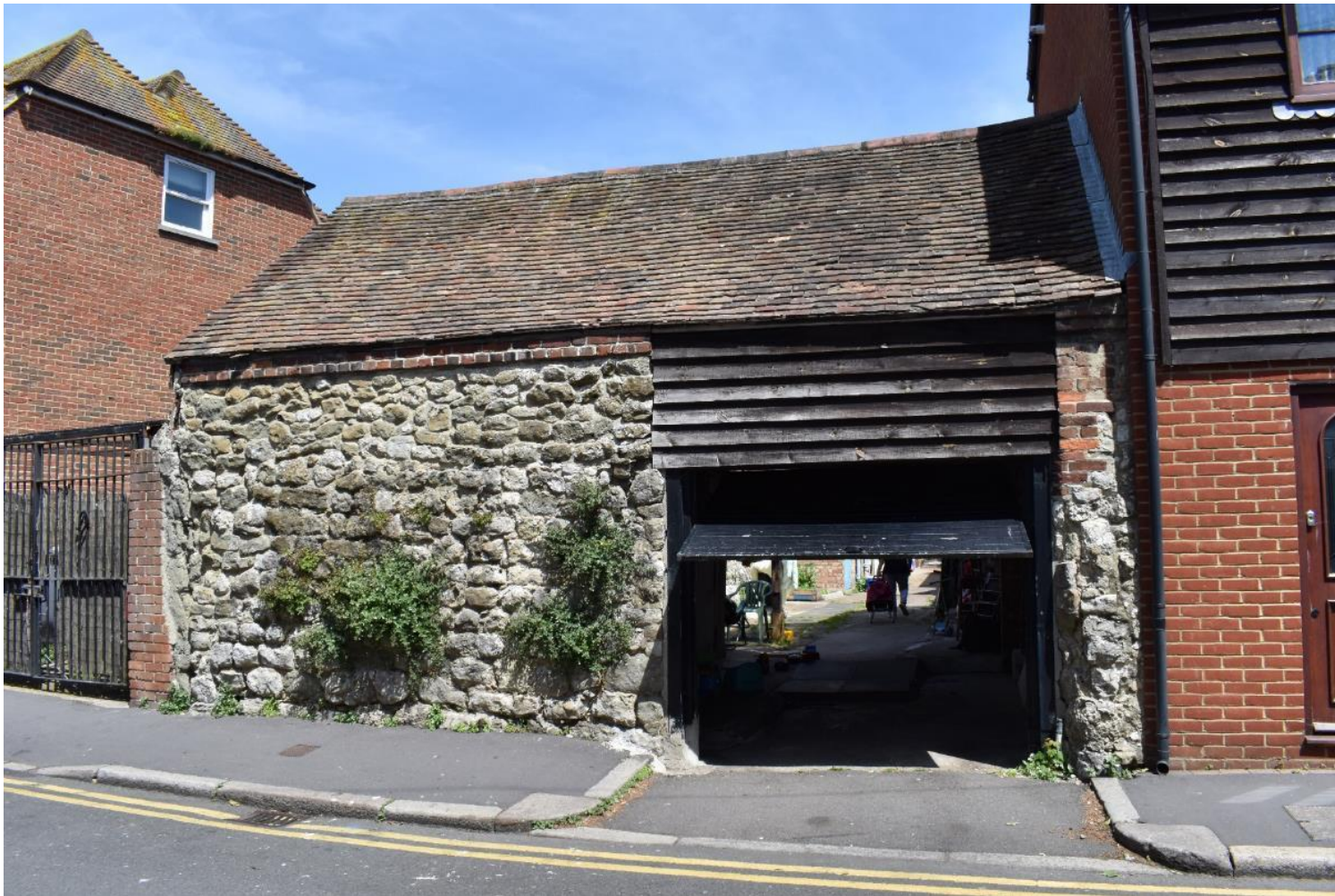
Plate 14: View of the southern boundary and garage entrance from Chapel Street (facing N)
