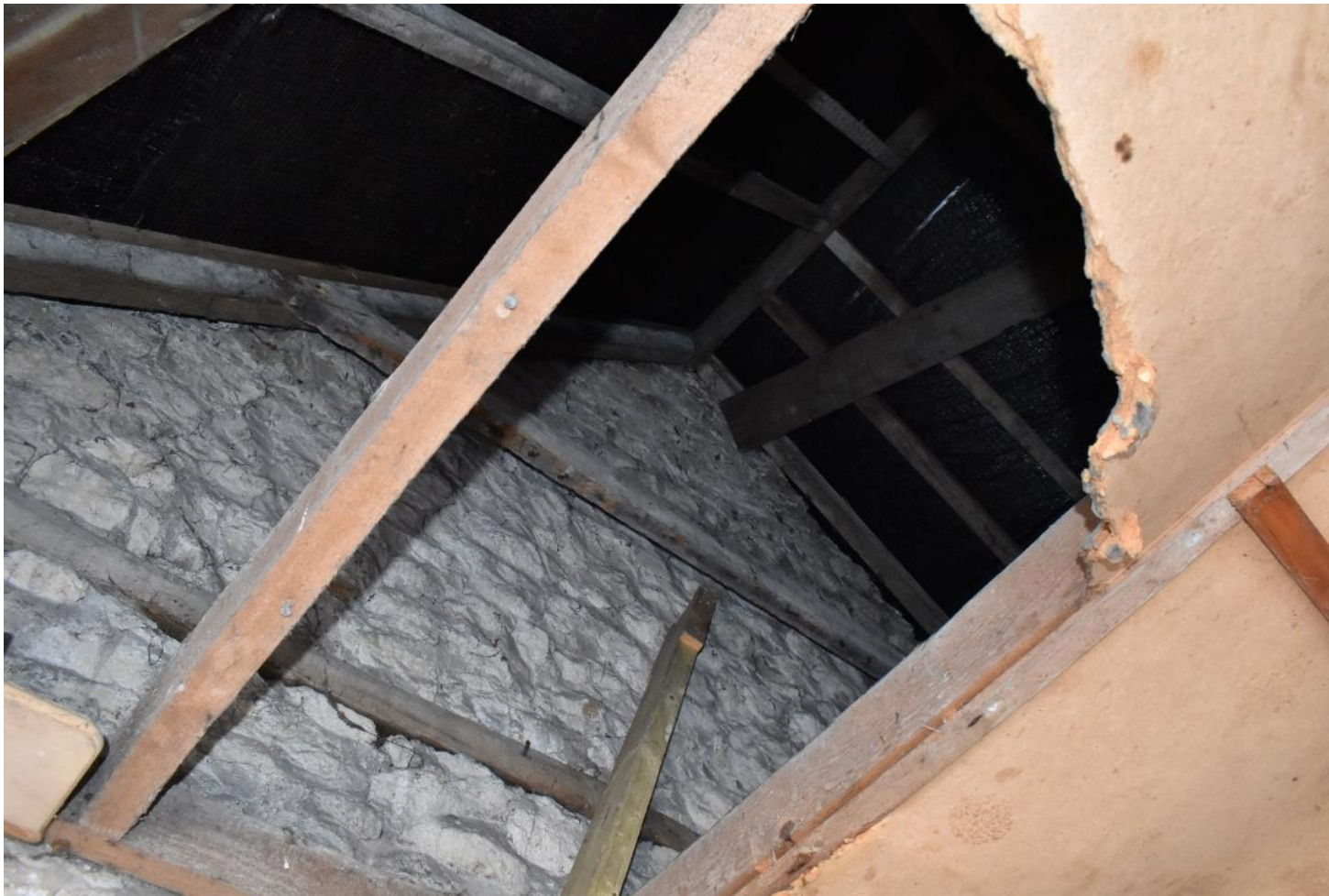
Plate 9: View of the eastern gable wall (facing E)
