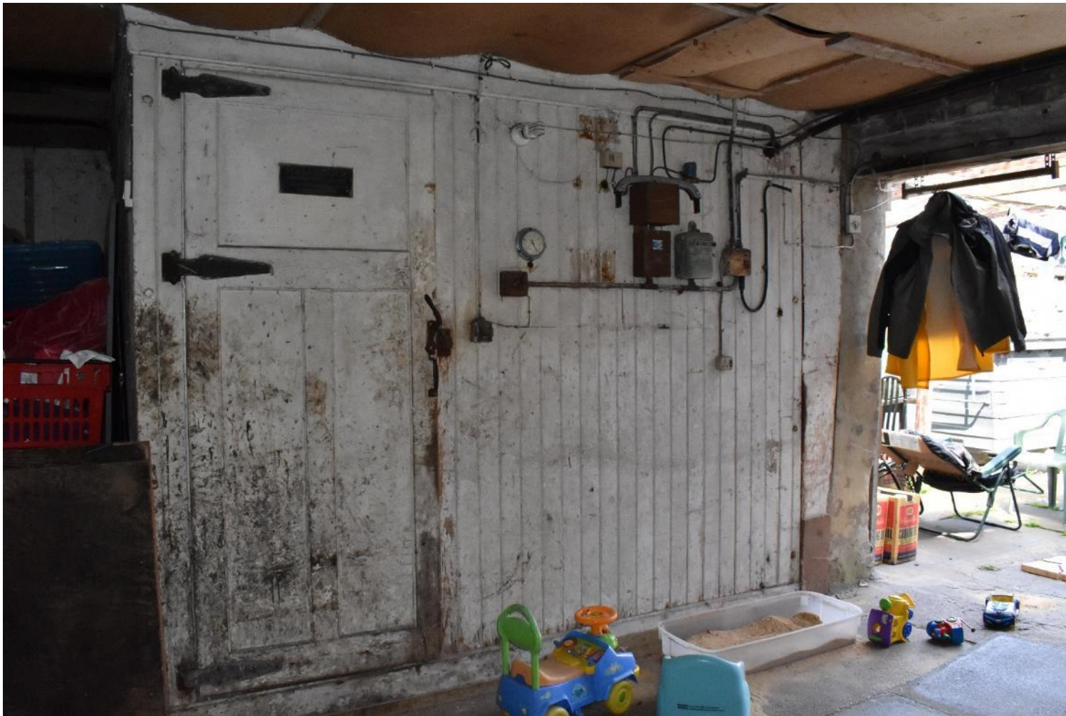
Plate 16: View of cold Store (facing W)
