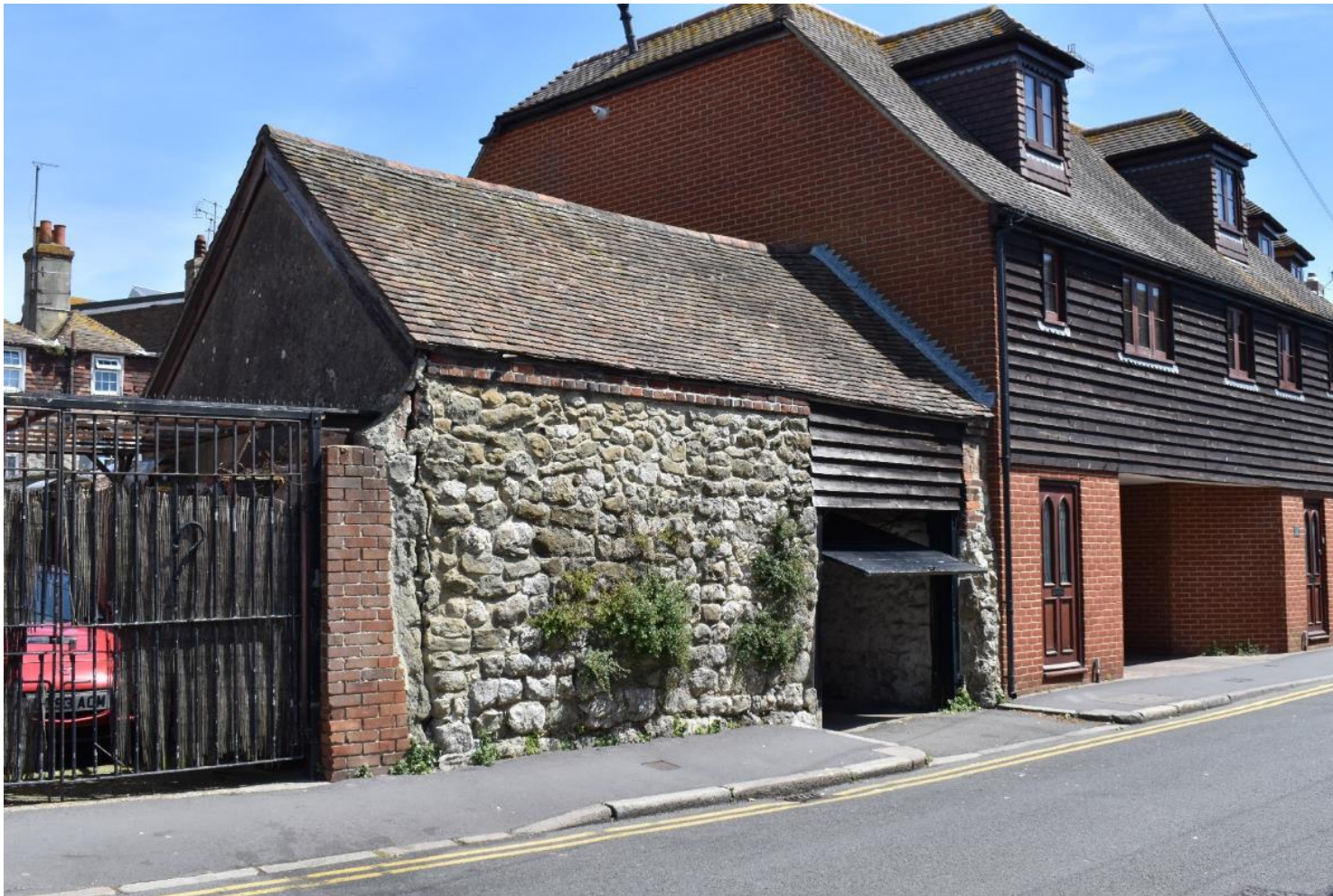
Plate 15: View of rear of PDA and western gable wall (facing NE)
