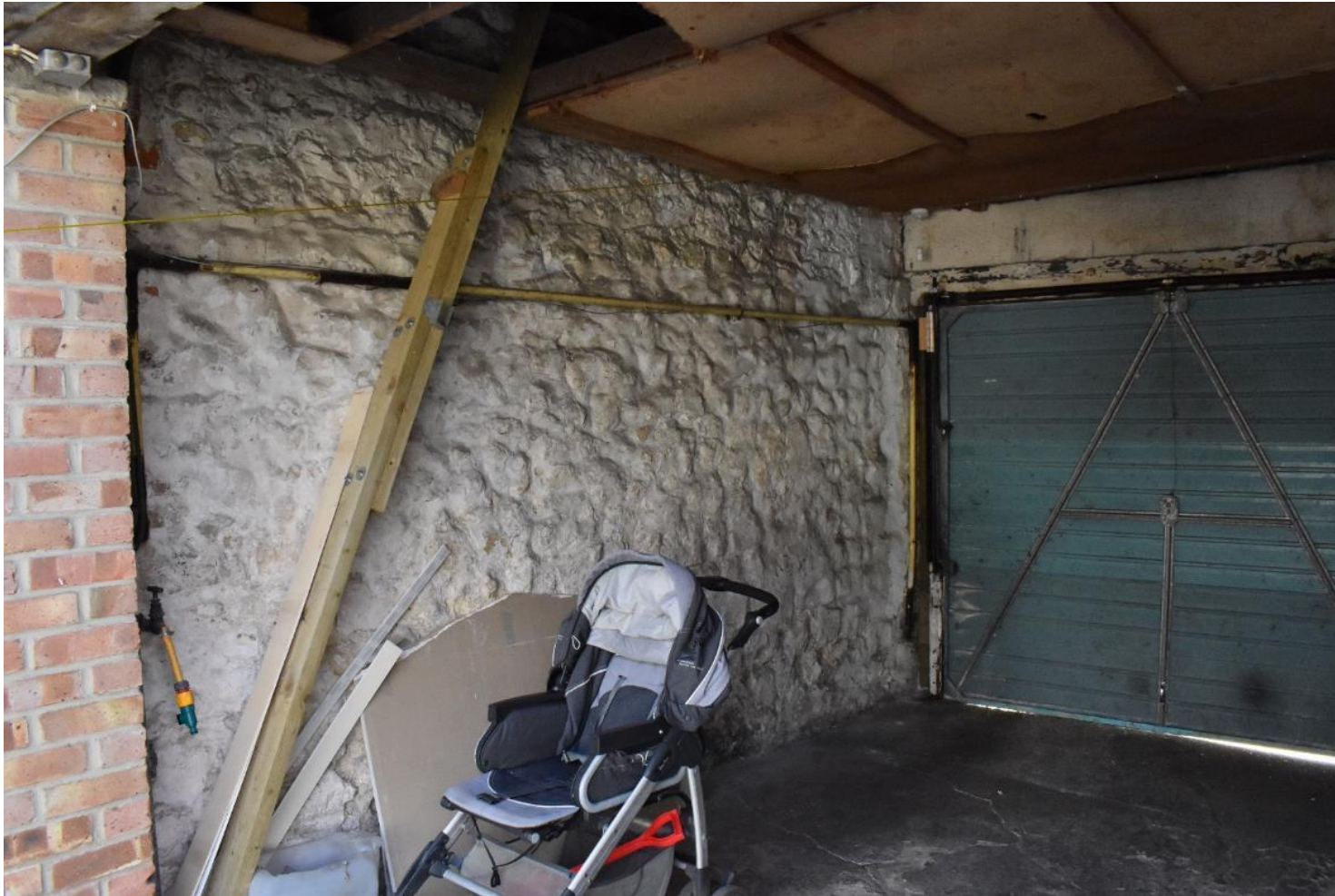
Plate 8: View of the east wall of the garage area (facing E).
